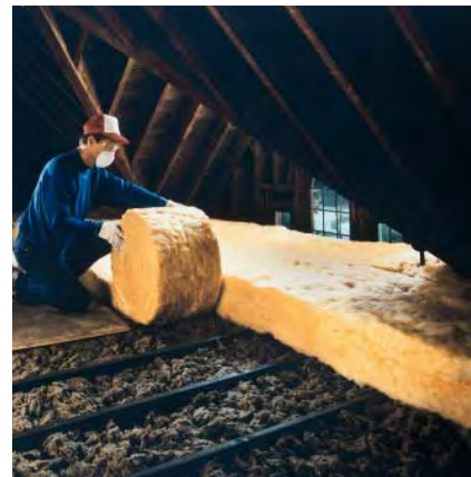
Layer fiberglass roll insulation perpendicular to the joists.
